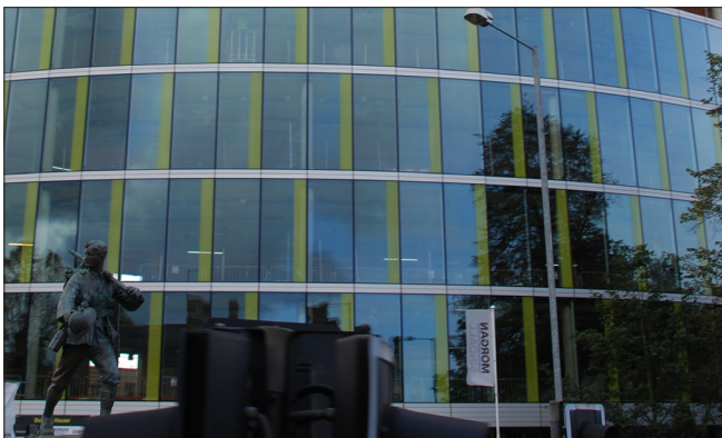
Figure 31: Curved glass curtain walling system on a modern office development in Cambridge.
